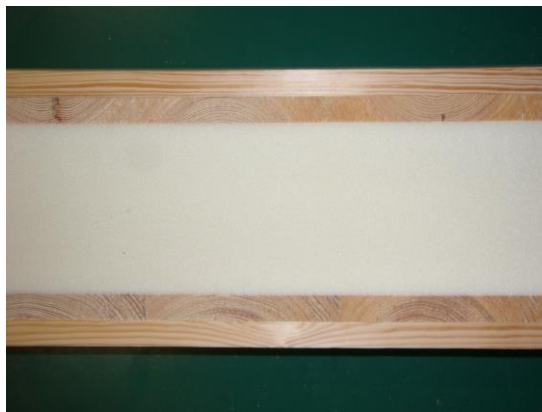
Figura 1: Example of the panel solution cross-section under development.
