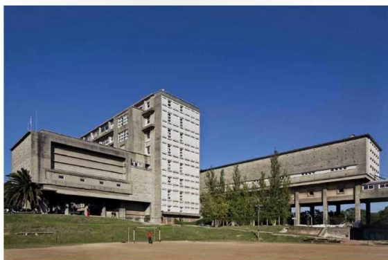
49901_110511_0170 General view from northeast
