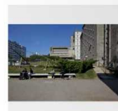
49901_110511_0190 View from the lateral street, pointing south
